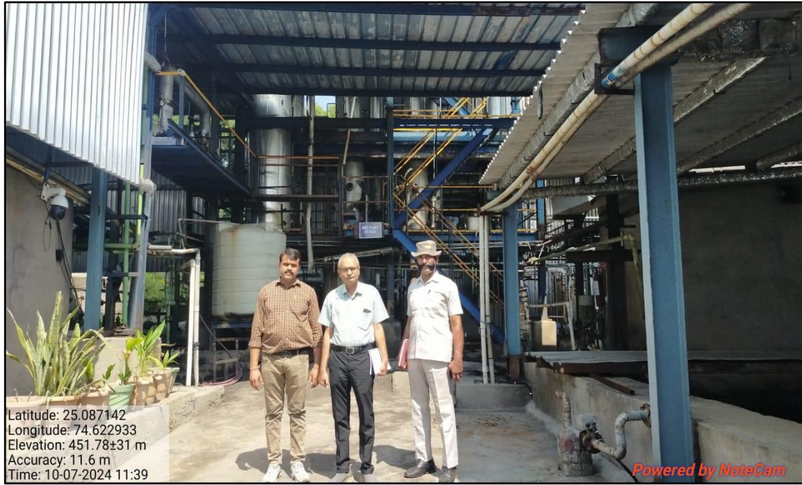
MEE and coal storage area.
